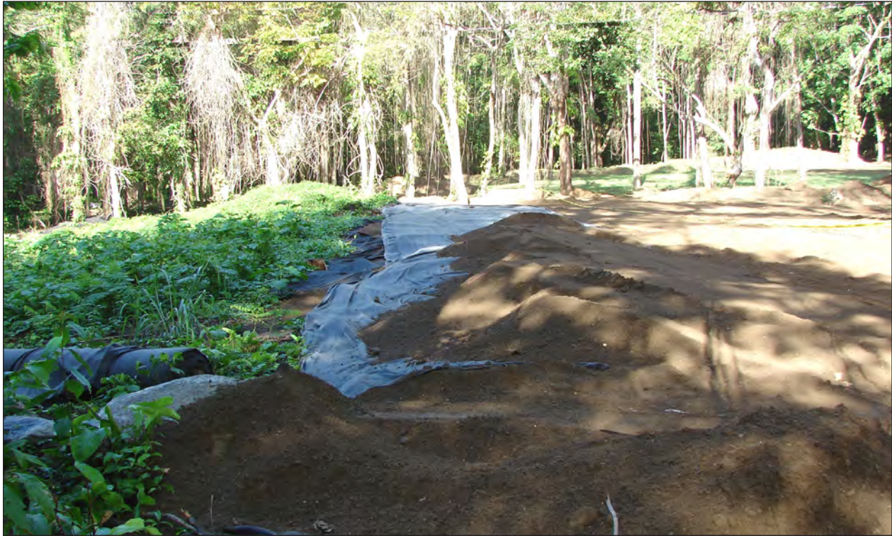
Figure 21. Midden Mound Covered with Geo-Textile Material
