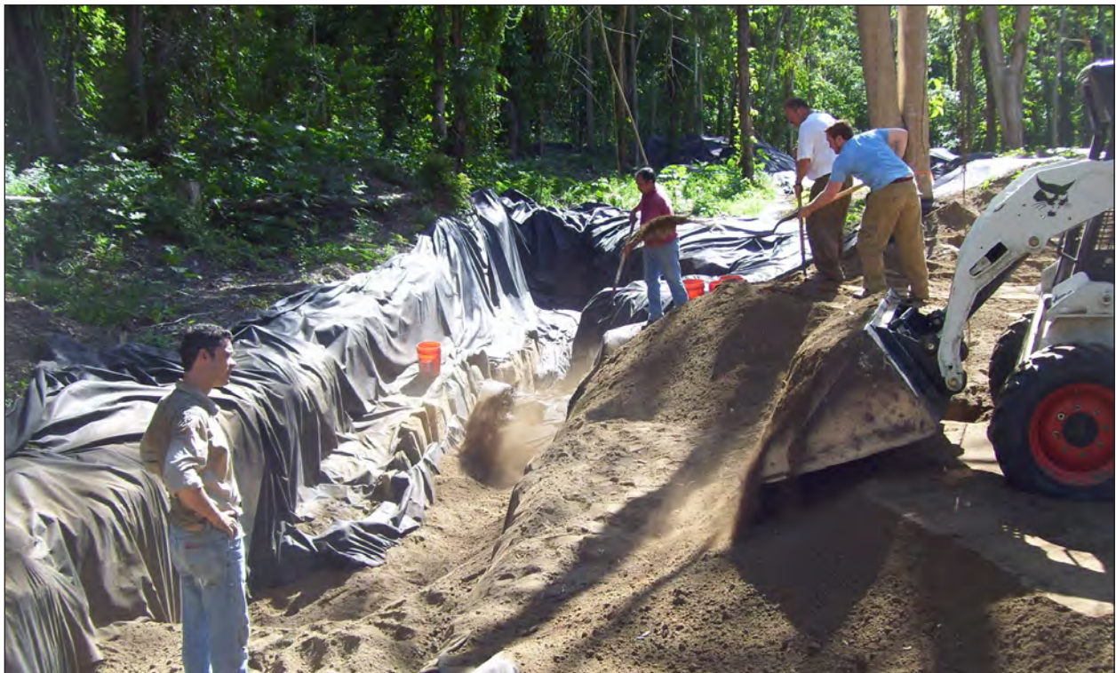
Figure 33. Shoveling Fill into West End of North Border Trench after Capping Stones with Cleaned Backdirt Fill
