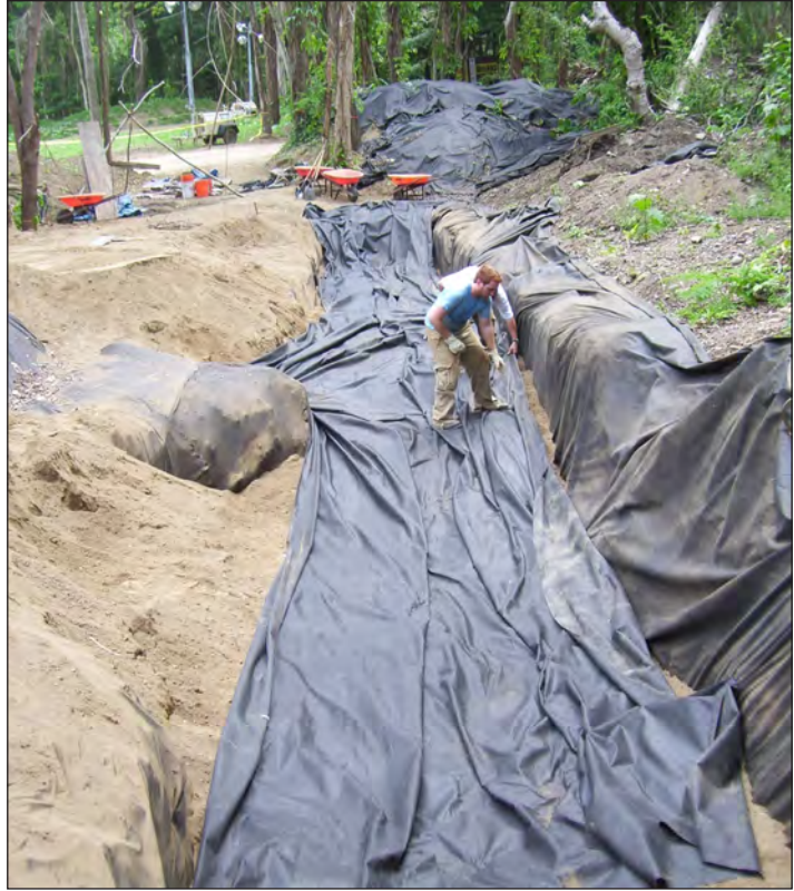
Figure 39. Final Filling of North Border Trench
