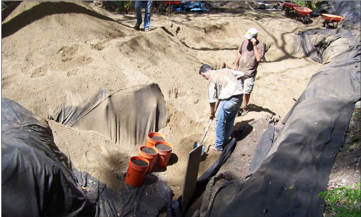
Figure 37. Leveling Alluvial Fill over the Capped Surface above the Petroglyph Stones
