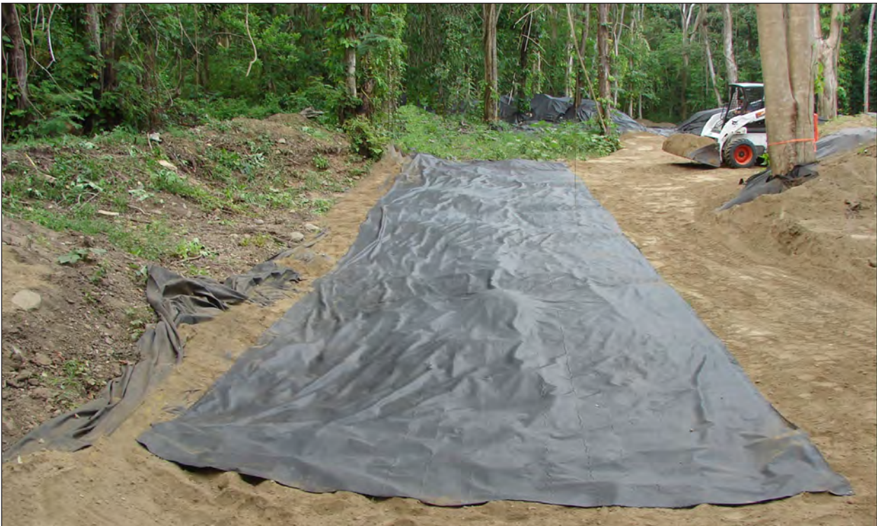
Figure 41. Placing a Geo-Textile Fabric Cover over the North Bordertrench Location
