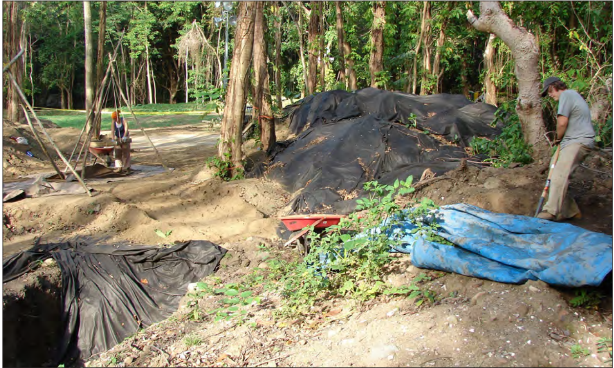
Figure 31. Placing Cleaned Fill Between Petroglyphs and Fabric
