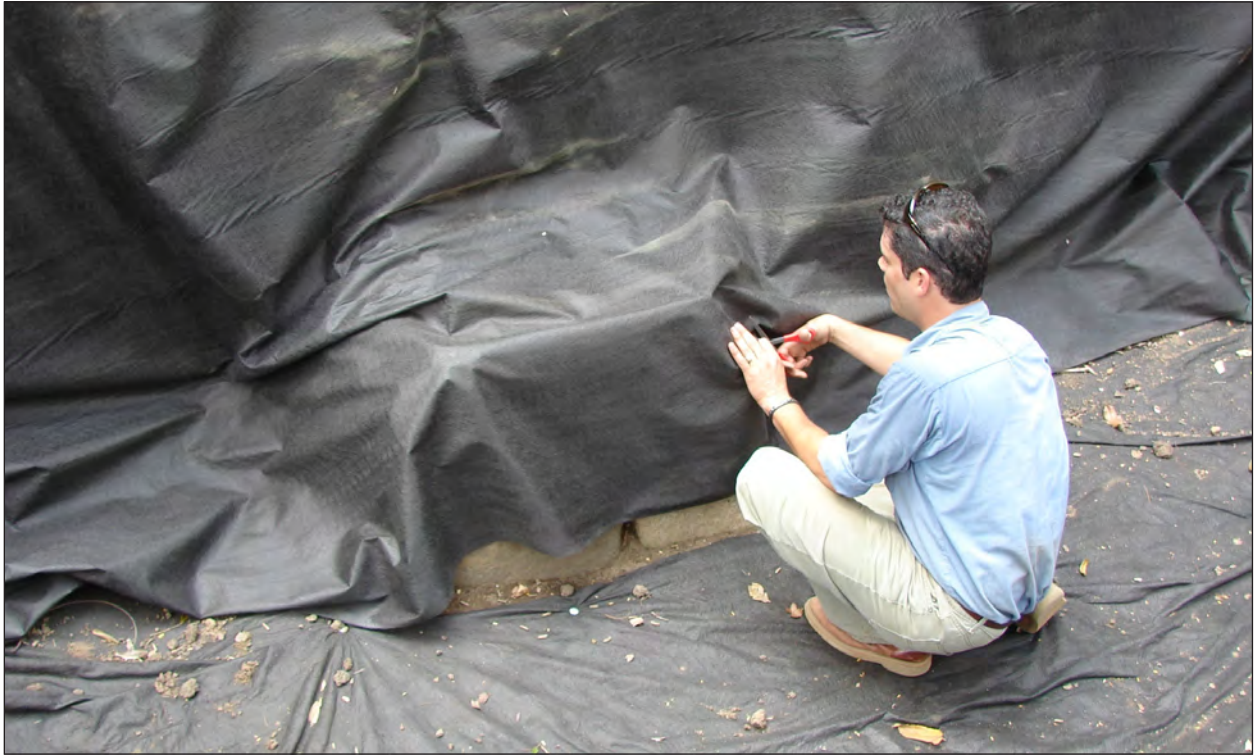
Figure 27. Securing Fabric Around Stones
