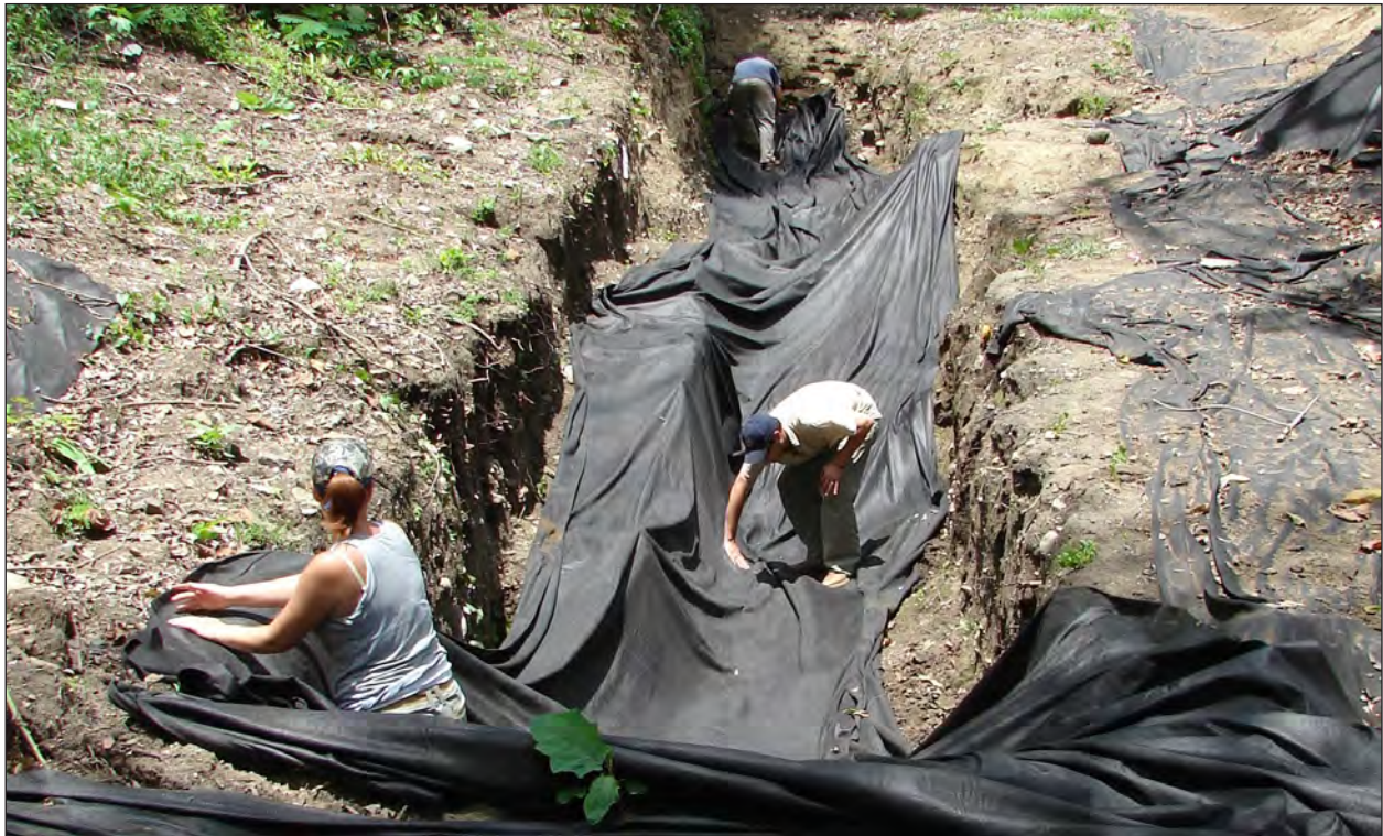
Figure 25. Placing Geo-Textile Fabric on North Border Trench Floor
