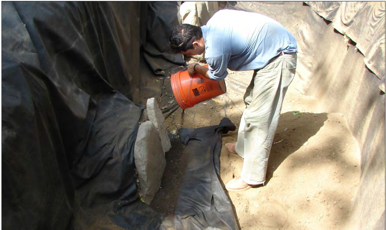
Figure 31. Placing Cleaned Fill Between Petroglyphs and Fabric
