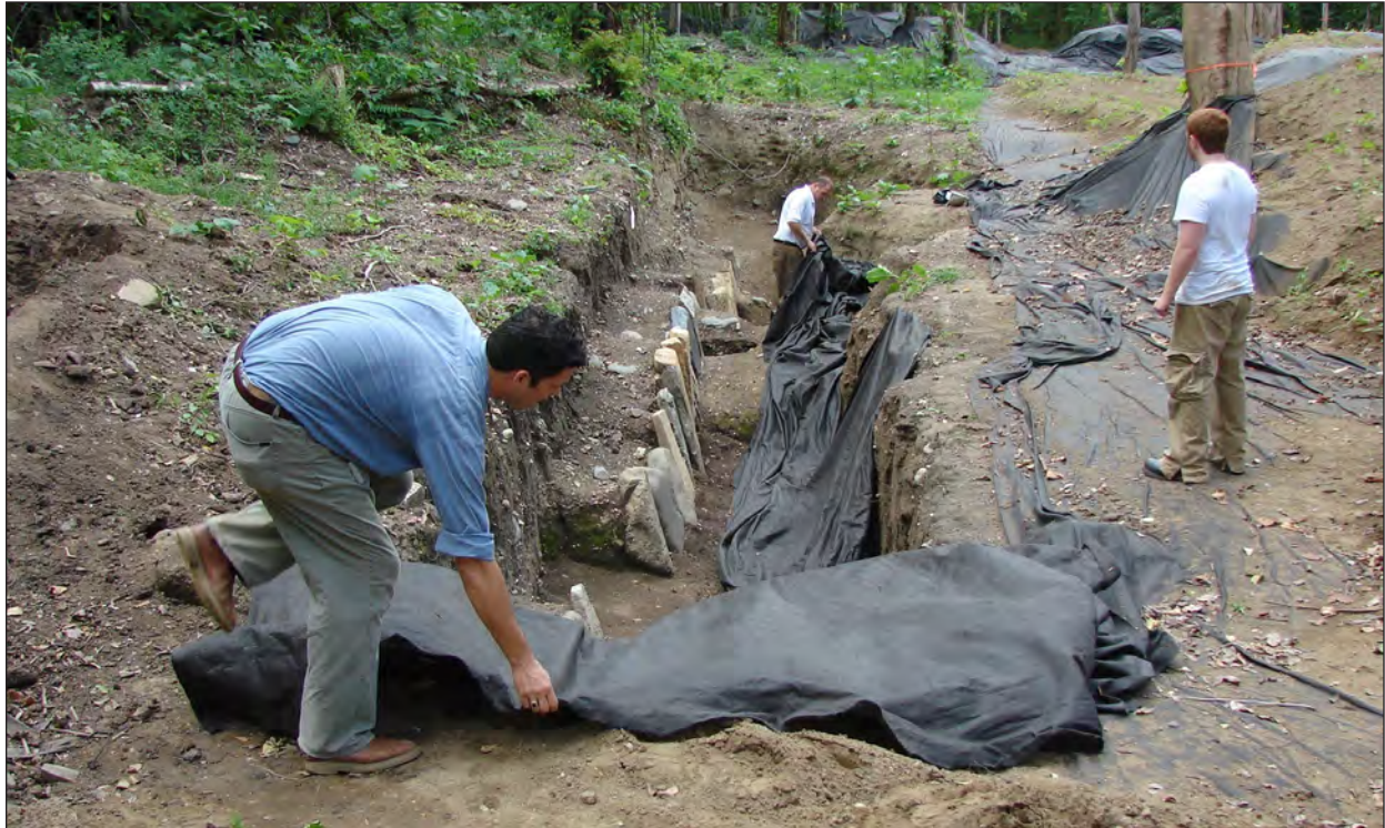
Figure 25. Placing Geo-Textile Fabric on North Border Trench Floor
