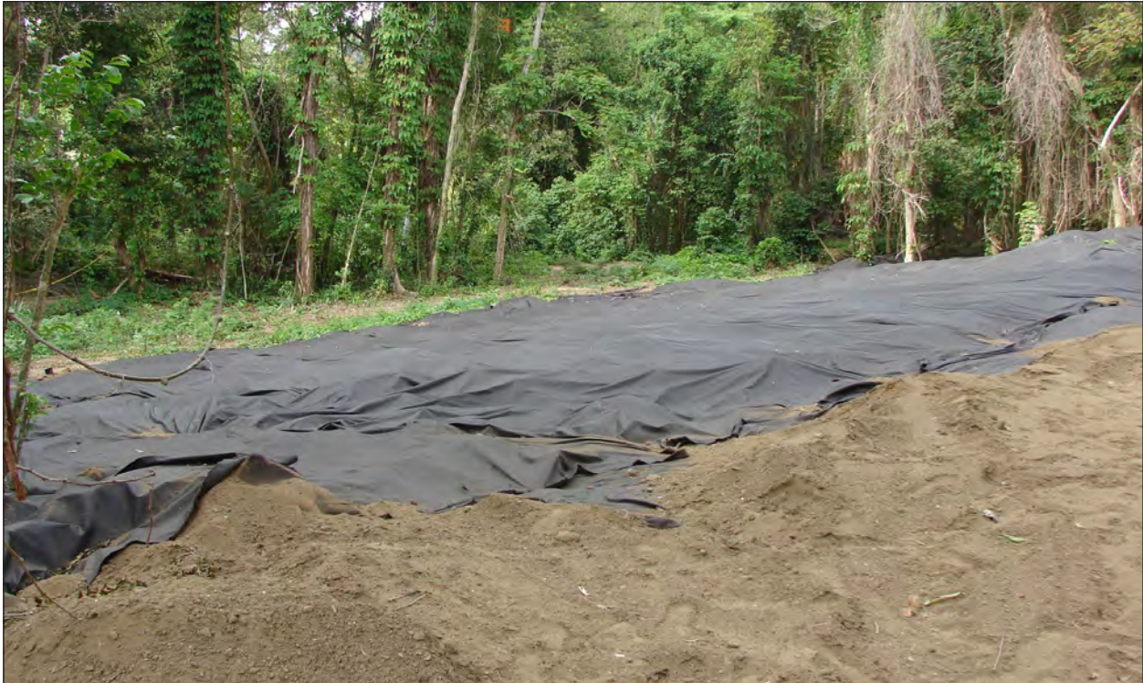
Figure 21. Midden Mound Covered with Geo-Textile Material
