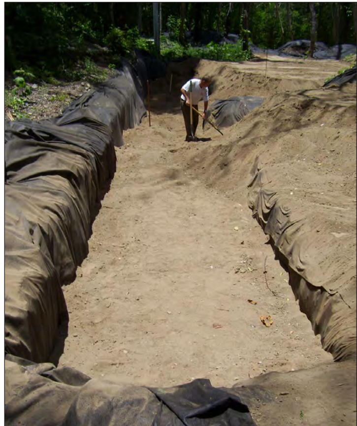
Figure 37. Leveling Alluvial Fill over the Capped Surface above the Petroglyph Stones
