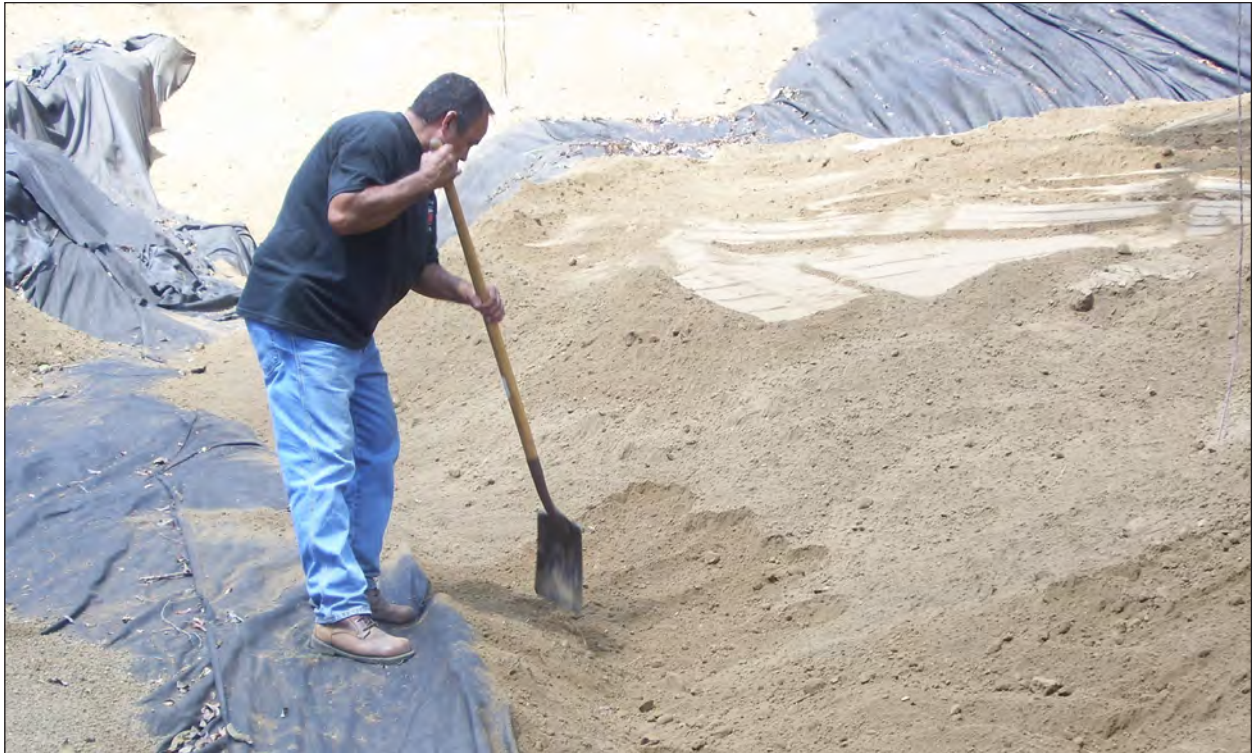
Figure 41. Placing a Geo-Textile Fabric Cover over the North Bordertrench Location
