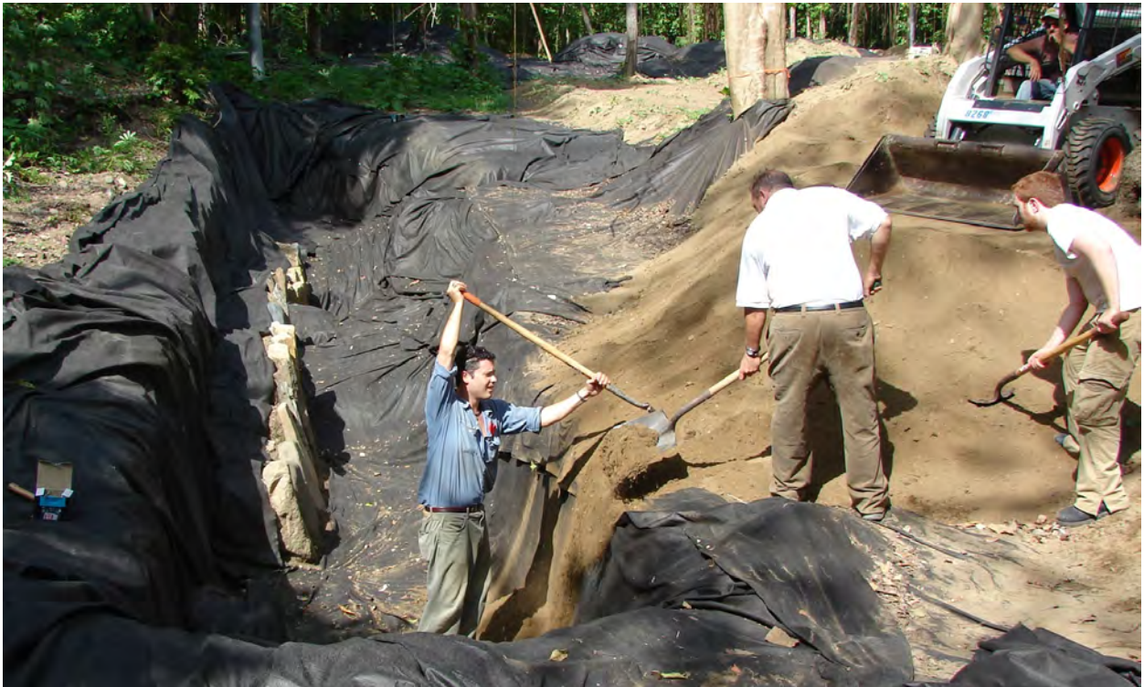
Figure 29. Shoveling Fill into Floor of North Border Trench
